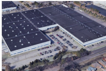
LRC PROPERTIES 4926 Southridge Blvd.
